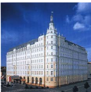
Silicone resin coating for the Kempinski hotel, Moscow
